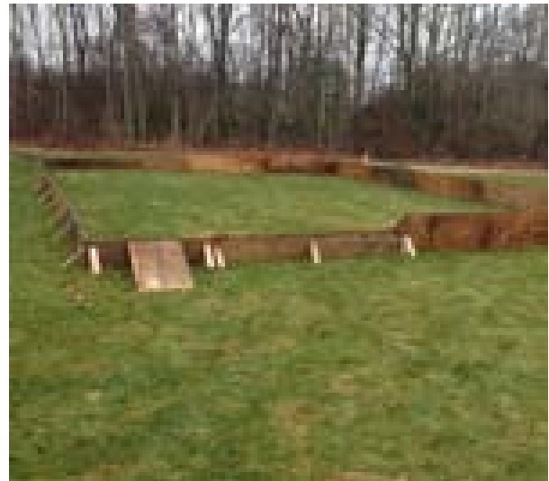
The frame for the 40 feet by 28 feet rink
